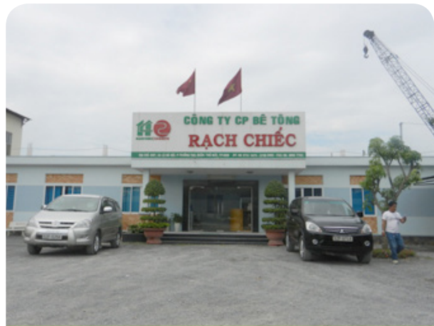
Rach Chiec concrete company
